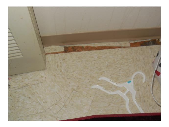
UPCS Inspectable Area: Units: Floors: Tiles are missing and/or broken. Level 1 (Level 2 or 3 for larger areas)
