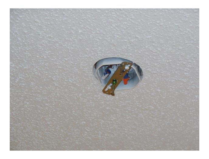
UPCS Inspectable Area: Units: Electrical: Covers: The cover is missing from a receptacle. Level 3
