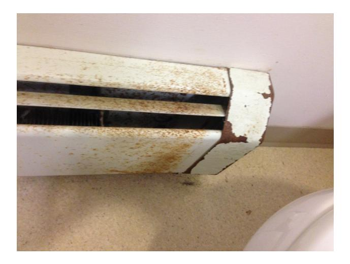
UPCS Inspectable Area: Units: HVAC: A radiator cover is rusted. Level 1
