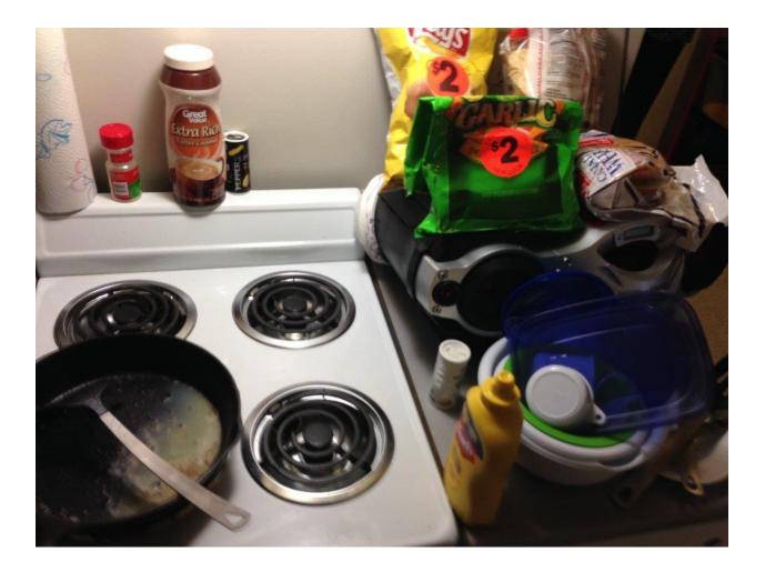
UPCS Inspectable Area: Health & Safety: Flammable Materials: Flammable items are being stored near the range. **Level 3**
