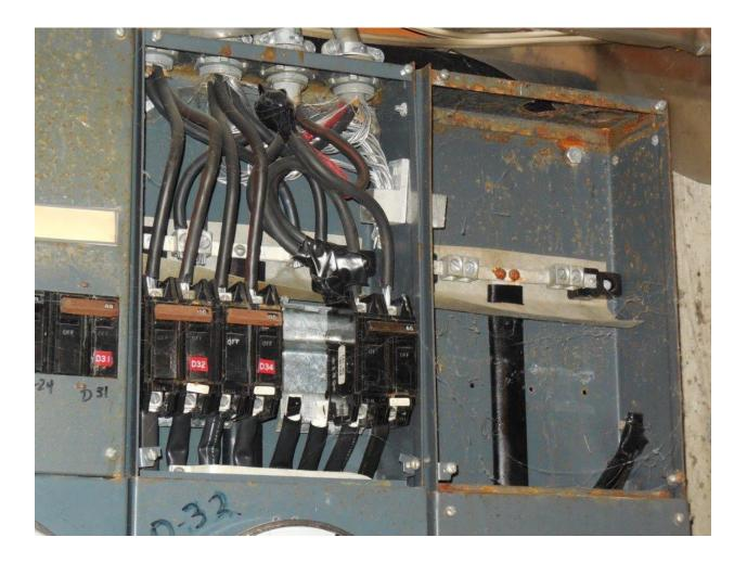
UPCS Inspectable Area: Health & Safety: Electrical Hazards: A panel is open and wires are exposed. **Level 3**
