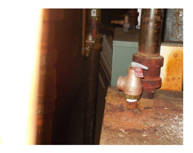
UPCS Inspectable Area: Building Systems: Domestic Water: The extension tube for the T&P valve does not extend within 18" of the floor. **Level 3**
