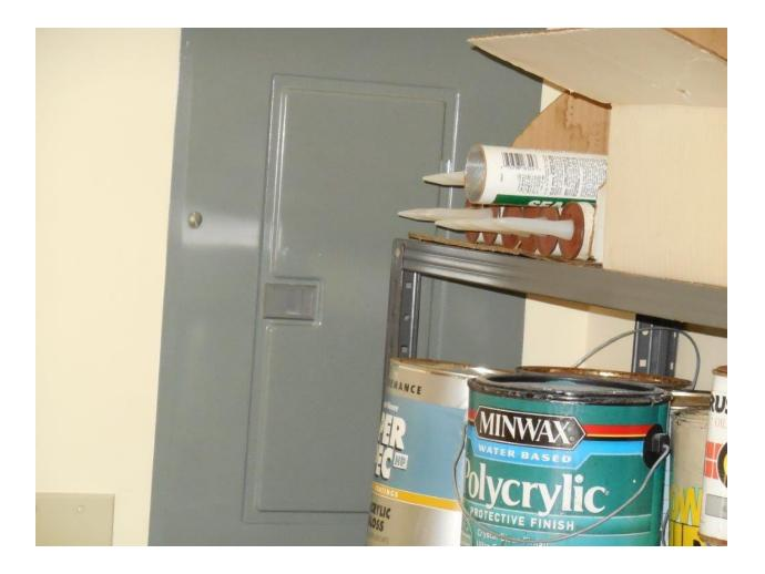
UPCS Inspectable Area: Units: Electrical: Panel: The electrical panel is blocked by a shelf. **Level 3**
