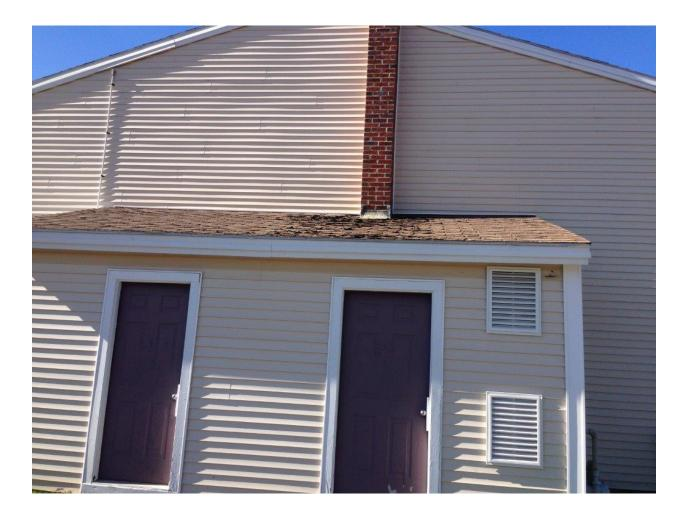
UPCS Inspectable Area: Building Exterior: Roofs: A portion of the roof is degraded. Level 1 (Level 2 or 3 for larger areas or more severe damage)
