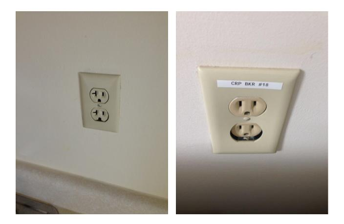
UPCS Inspectable Area: Units: Electrical: Covers: The receptacle is damaged. Level 3
