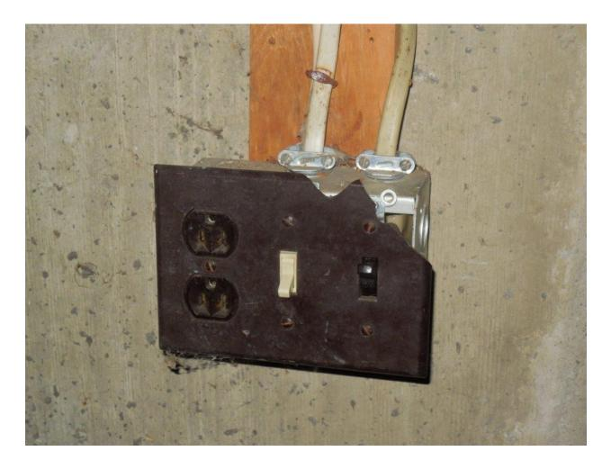
UPCS Inspectable Area: Units: Electrical: Covers: The receptacle cover is damaged. Level 3
