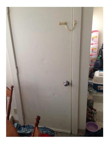
UPCS Inspectable Area: Health & Safety: Emergency/Fire Exits: An auxiliary lock has been installed above 48" from the finished floor. **Level 3**
