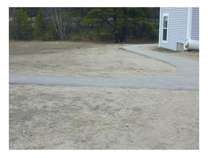
UPCS Inspectable Area: Site: Grounds: A large area of the site is eroded and has caused a degraded surface. Level 2
