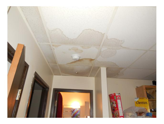
UPCS Inspectable Area: Units: Celing: Ceiling tiles are stained, bulging and sagging. Level 3 (Level 1 or 2 for smaller stains that do not damage the ceiling)
