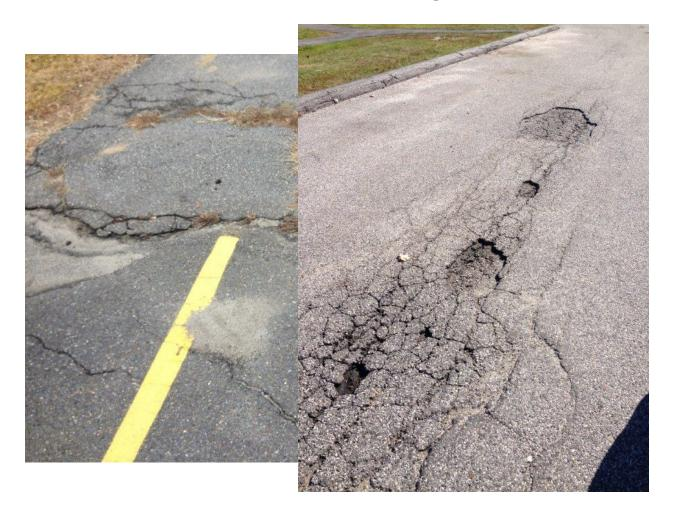
UPCS Inspectable Area: Site: Parking Lots/Driveways/ Roads: A large area of pavement has large cracks, heaving, potholes and settling. Level 2 (Level 3 for more widespread, Level 1 for less)
