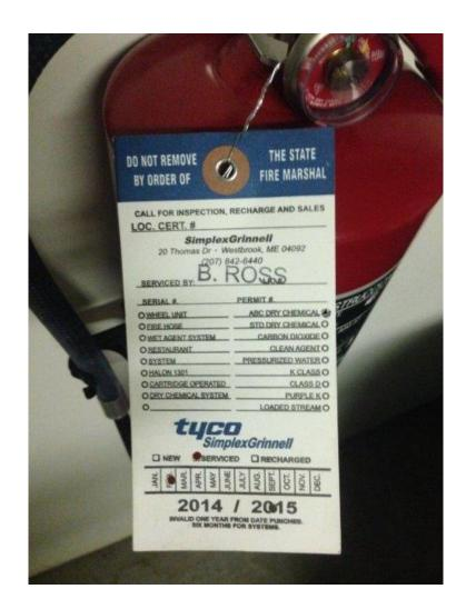
UPCS Inspectable Area: Building Systems: Fire Protection: A fire extinguisher is expired. Level 1 (Level 3 if throughout the building)
