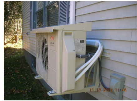
Outdoor component must be protected by a rain cap if located under a drip edge.
