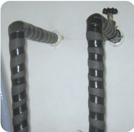
Secure seams with tape
