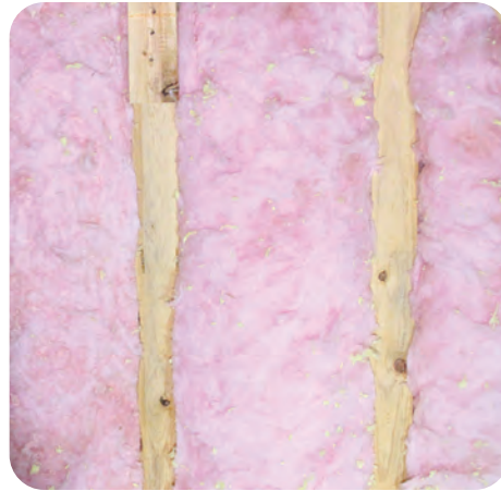
2. Cut batts for exact fit
