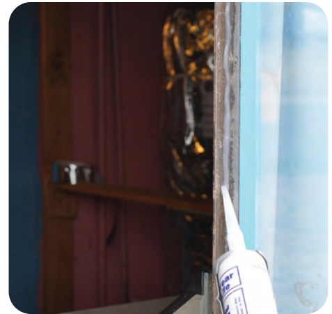
4. Run interior bead of caulk
