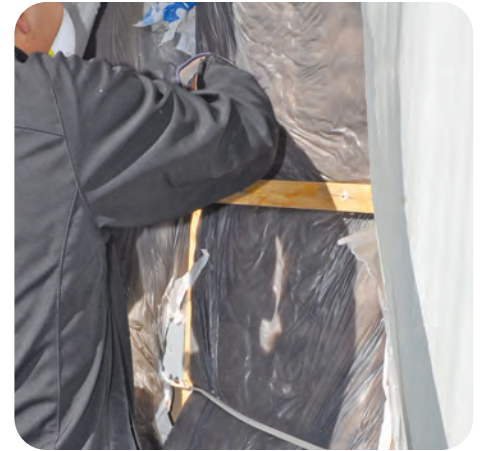
7. Gently tug batt into place and tuck remaining batt under lower belt rail and fit down to bottom of cavity with minimal compression
