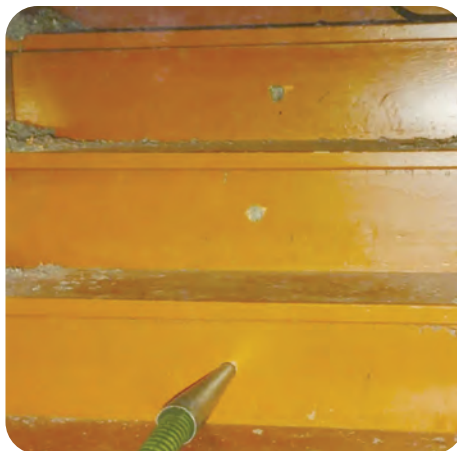
11. If backside of stairs is sealed, blow insulation into cavity behind stairs
