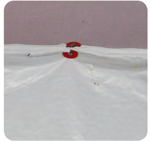
3. Seal seams of belly wrap
