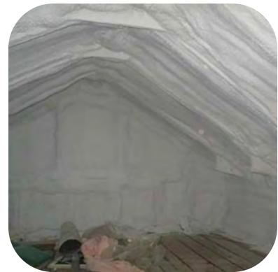
Unvented Roof Deck Application
