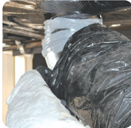
2. Pull insulation over hard connections as needed
