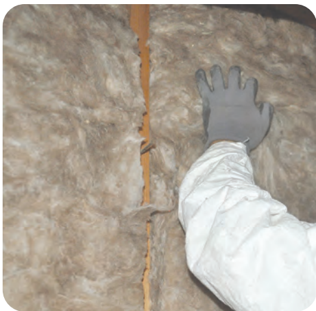
3. Install batts with minimal compression
