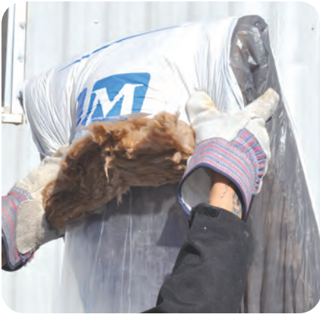
5. Fold batt over end of insulation stuffer
