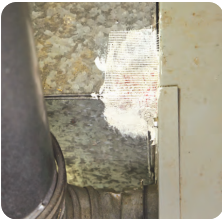
B-4. Push fiberglass mesh into the mastic
