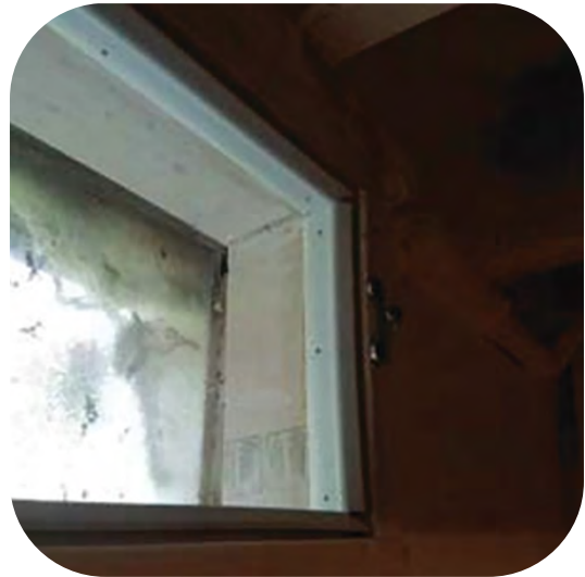
Weatherstrip around window and basement door cavities to create air seal
