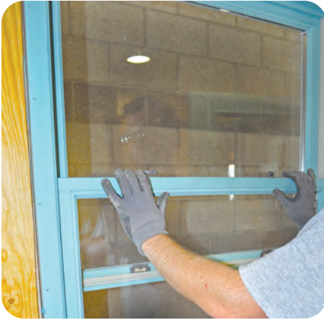
7. Ensure window is operational
