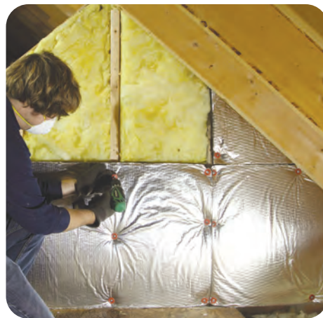
4. Install backing material
