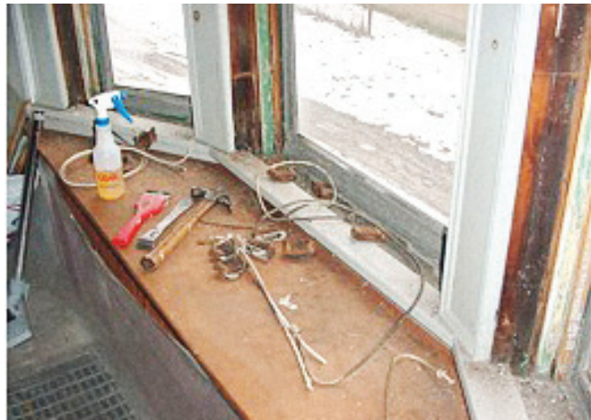
FIGURE 11.9 Window after removal of sash weights.
