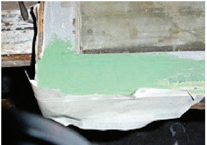
FIGURE 11.10 Rebuild damaged sash with filler or putty.
