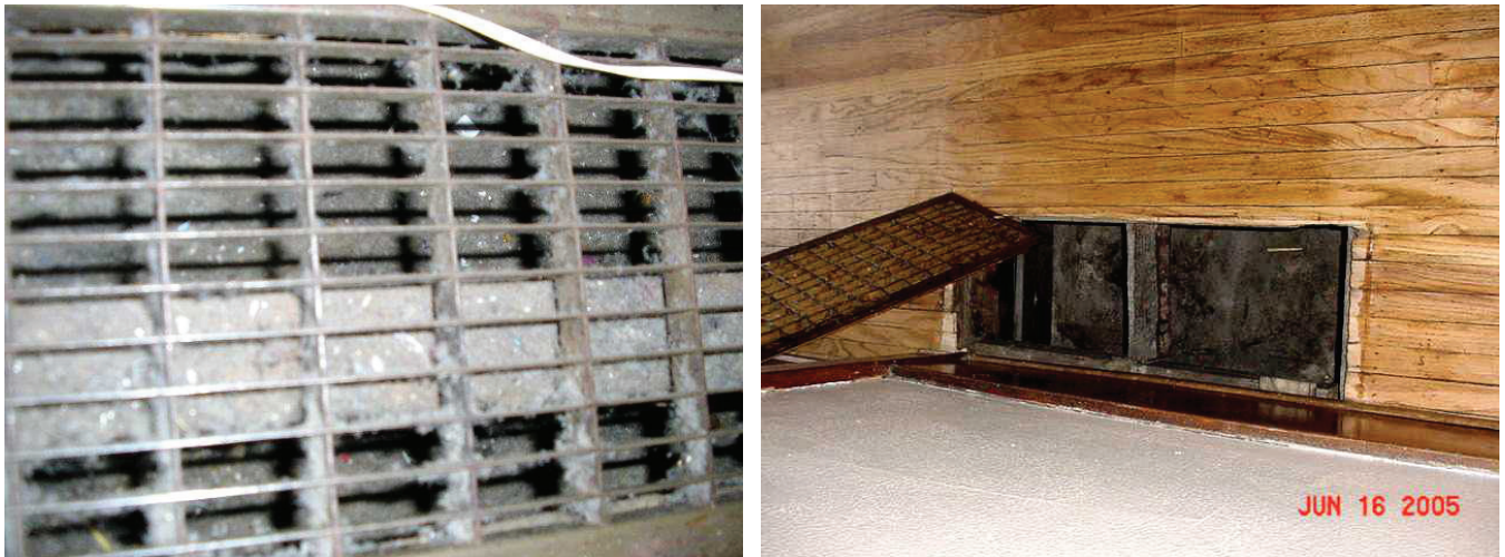
Figure 11.24 Air vent before and after cleaning.
