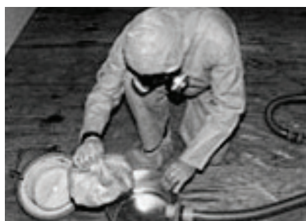
b) Disconnect Vacuum Bag From Hose Inlet
