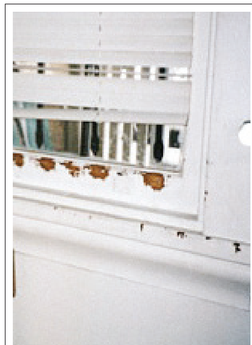
FIGURE 5.8 Chewable surface: teeth marks on window sill.
