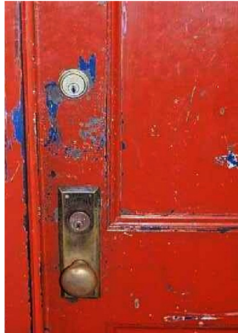
FIGURE 1.3 Paint deterioration.
